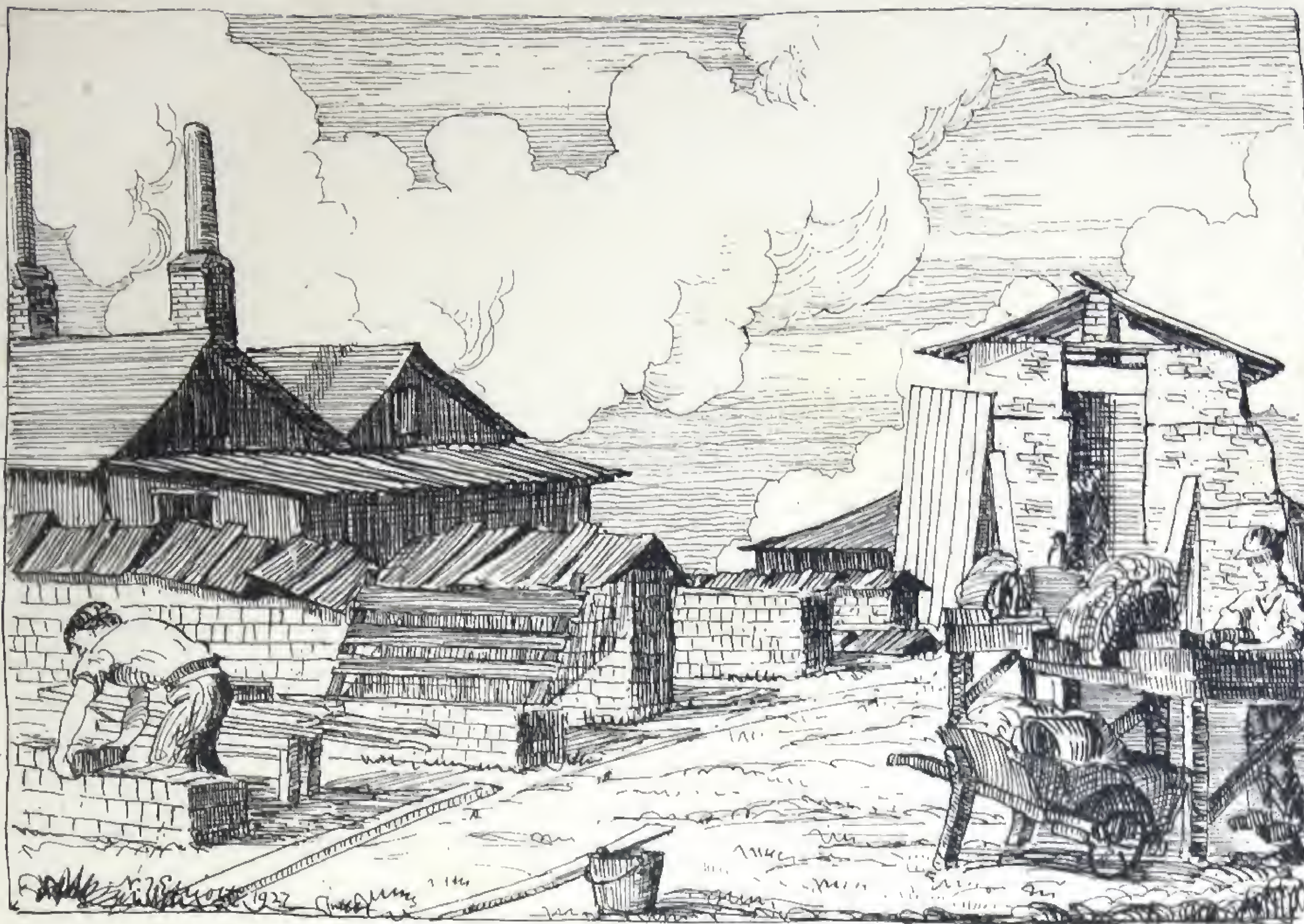
General View of Old Style Brick Works
