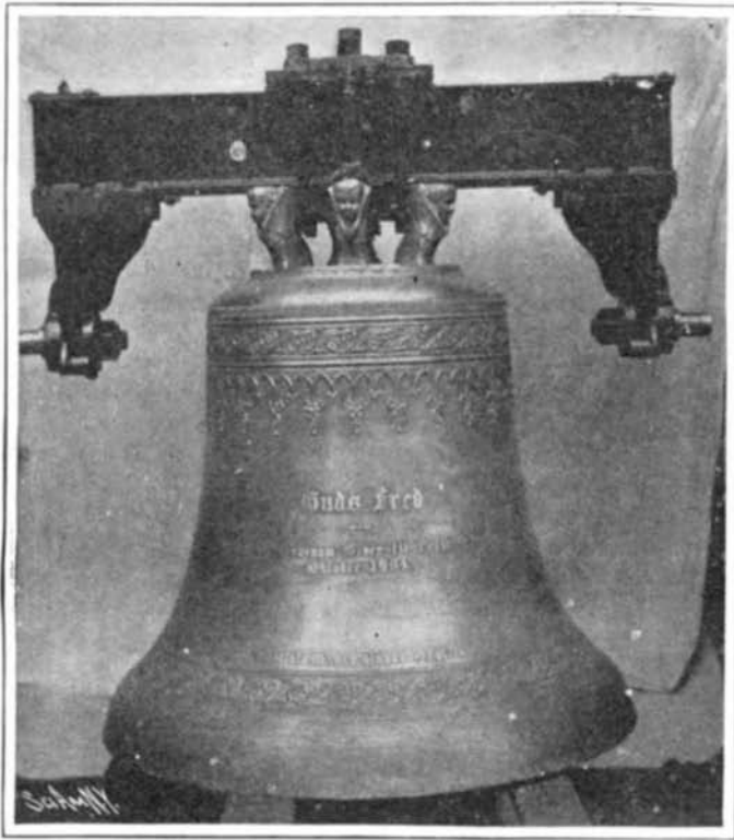
The Bell for the Free Harbor Church at Copenhagen, Showing the Balanced Suspension System.
