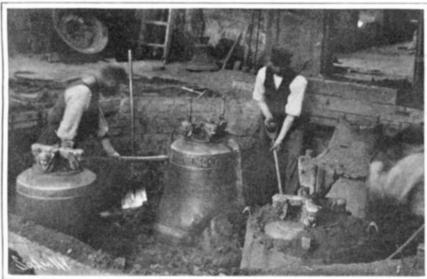
Digging Out the Cast Bells.
