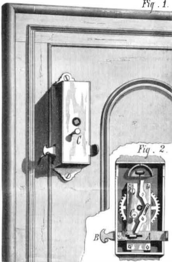
When it is desired to hold the alarm out of action, a pin, C, is pushed inward so as to prevent the movement of the escapement arm.
